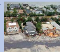
During Superstorm Sandy in 2012, storm surges brought water inland and flooded the coastline of New Jersey. Source: U.S. Air Force/Master Sgt Mark C. Olsen.
