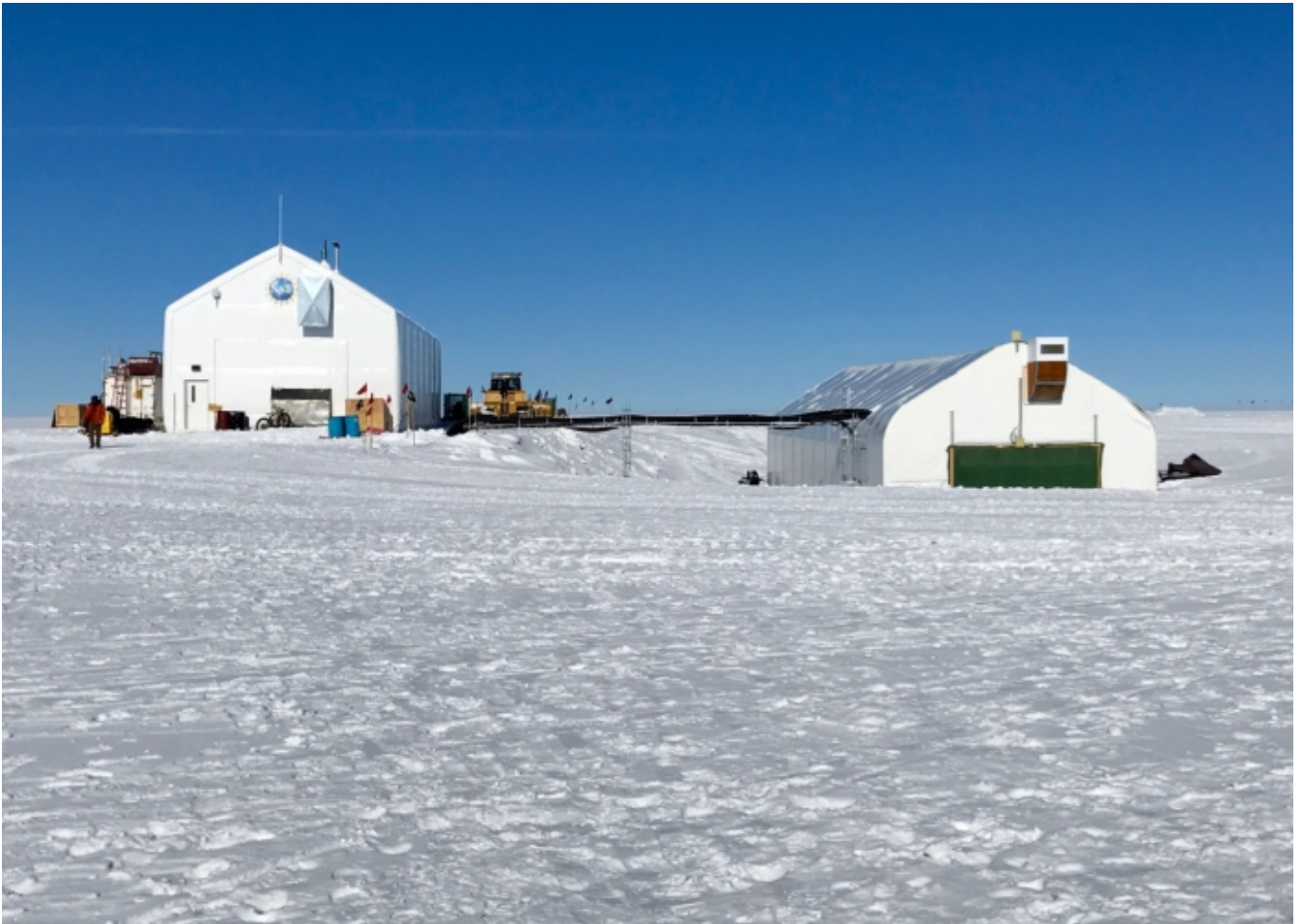
A new mobile garage (on left) has been constructed at Summit Station. The garage sits on a mobile sled-like base that allows the garage to be periodically towed into a new position to combat surrounding snow accumulation and drift. The old garage (on right) sits below the horizon and will be deconstructed and removed from station beginning in 2018. Photo courtesy of Jennifer Mercer.
