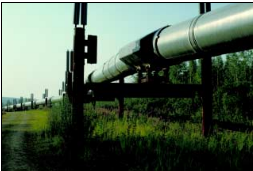
Figure 5-6. The Trans-Alaska Pipeline is designed to keep permafrost frozen by the use of thermosiphons. Permafrost is warming in interior Alaska, where this picture was taken (photo by L. Hamilton).
