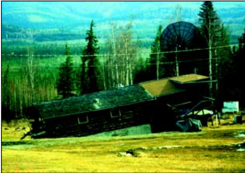
Figure 5-5. Structures can be dramatically affected if the underlying ice-rich permafrost thaws (photo by L. Hinzman).
