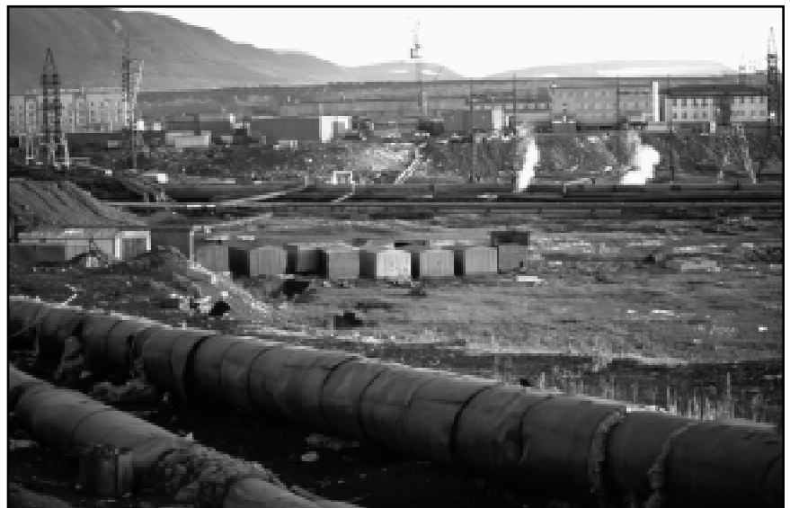
Ore-processing and other industrial facilities at Norilsk, Russia in August 1995. The metallurgical complex of Norilsk at 69°N in northern Siberia is the largest point source of atmospheric pollution in the Arctic (photograph by Henry Huntington).
